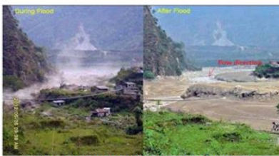
Seti Flood in Kharapani (2012) Photo: (Kattel, 2014)
